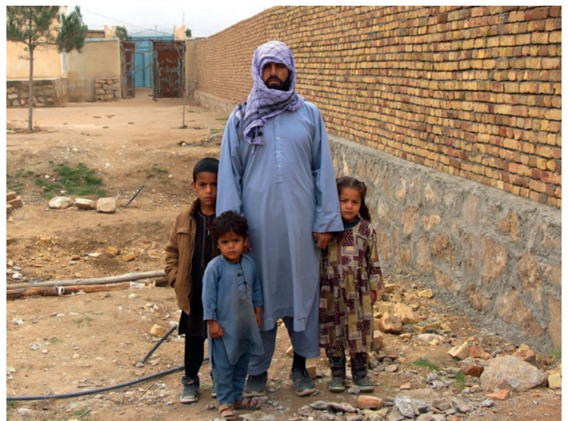
Shaista and his children proudly stand next to their newly repaired boundary wall in Karkar village, Pul-e-Khumri, Baghlan province
