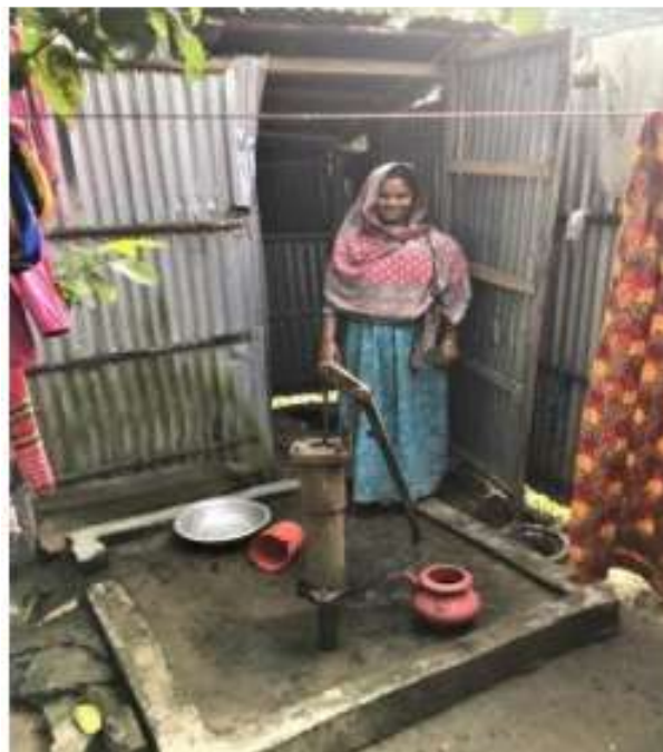
Examples of a newly constructed tube well and latrine in an ALO household during the project period
