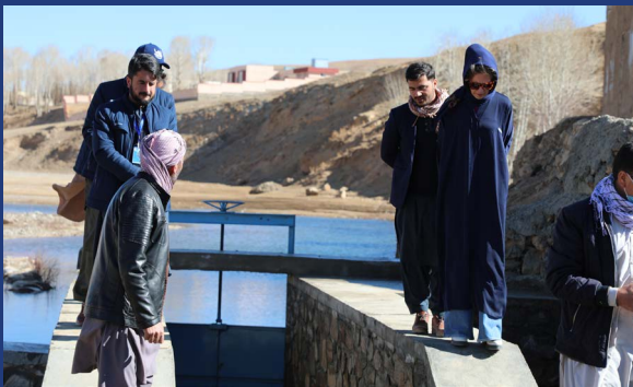
Ghor: Improving irrigation infrastructure to increase farmers' productivity and income and reduce disputes between farmers over water usage.
