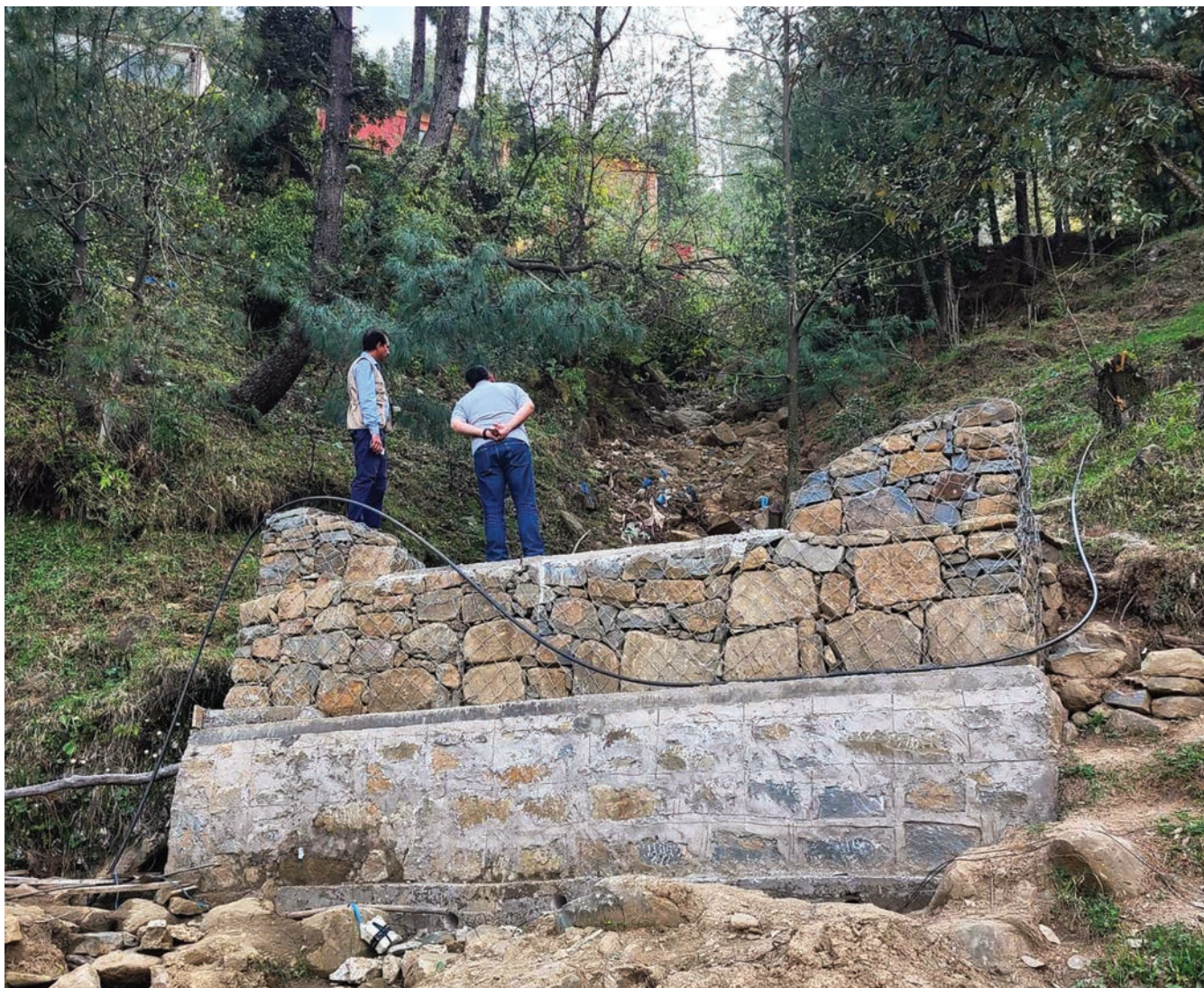
Islamic Relief worked with the local community to build this check dam above a village in AJK, where flash floods had previously destroyed four homes and a mosque. The dam stood firm in the 2022 monsoon, protecting 20–25 houses from harm
