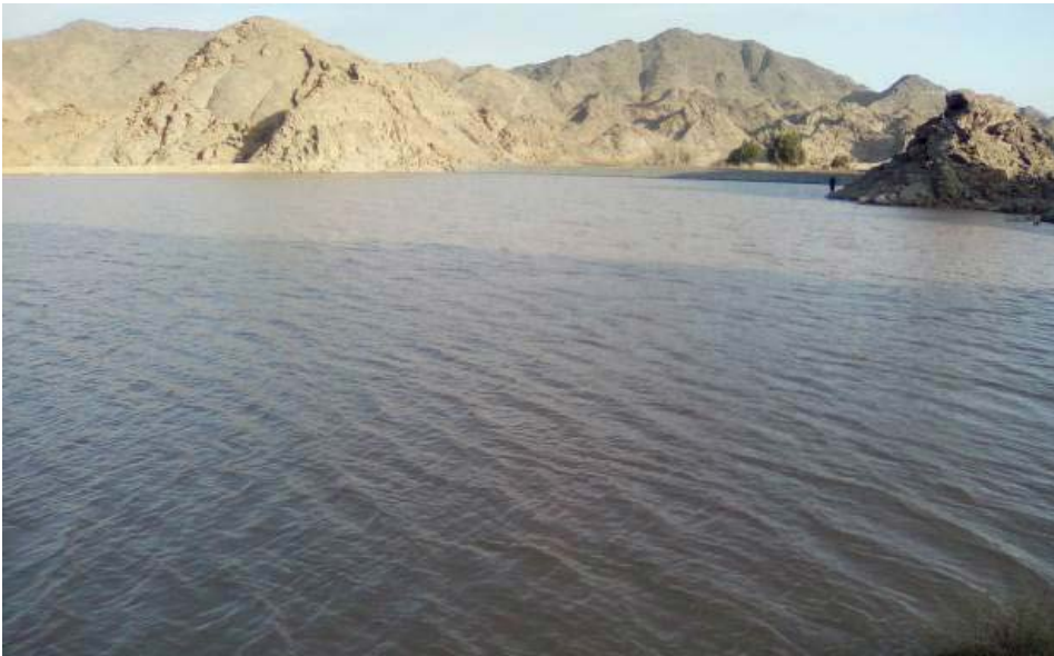
Water reservoir constructed in Chagai, Balochistan under Drought Resilience Agricultural Modeling DRAM Project.
