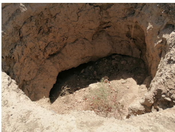
Dried up Karez (underground irrigation tunnels) in Purana Mian Khanzai
